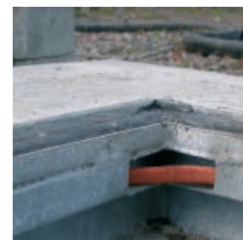
3. Heating cable - protects against frost and ice damage.
