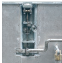
2. Copenhagen lock - mortise lock system - a simple and functional locking mechanism combined with a bracket for panic opening.
