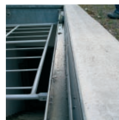
5. Rubber seal prevents penetration by water.
